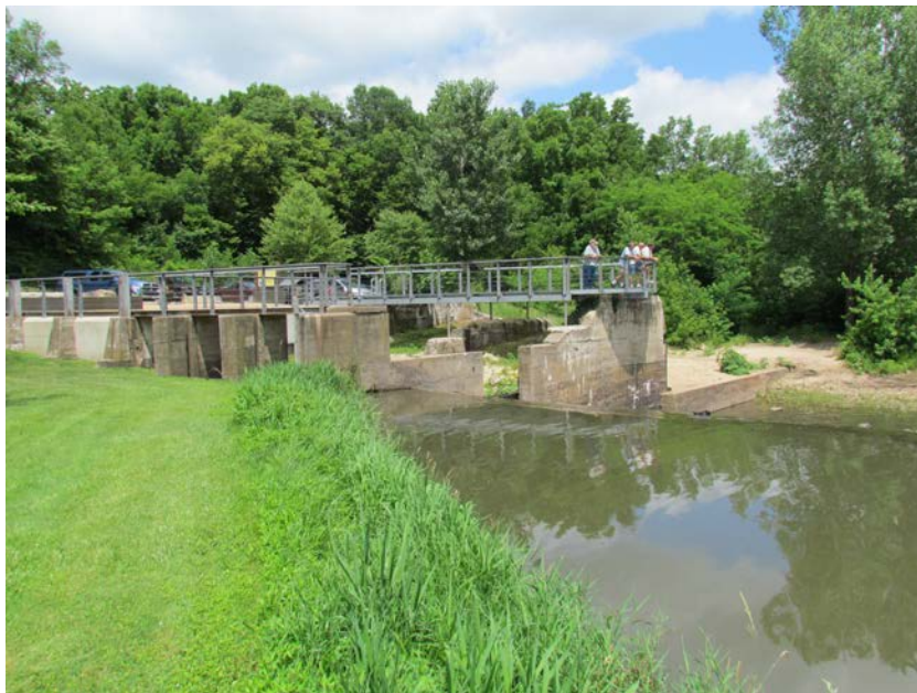
Figure 12. Former race walls and observation deck at the Monticello Electric Company Dam (site 53-00900), near Monticello, Iowa, facing northeast. Photograph by Richard Carlson, June 23, 2016.
