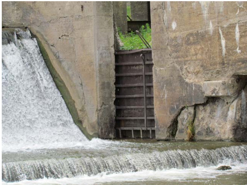
Figure 7. Sluice gate in the race wall at the Monticello Electric Company Dam (site 53-00900), near Monticello, Iowa, facing northwest. Photograph by Richard Carlson, June 23, 2016.
