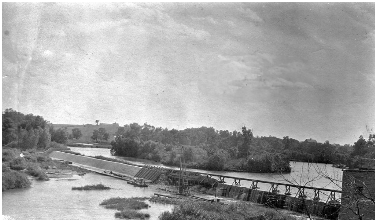
Figure 15. Historical photograph of the construction of the Monticello Electric Company Dam (site 53-00900), near Monticello, Iowa, facing southwest. The photograph is mistakenly dated to 1902, but it more likely dates to late summer or fall of 1913, shortly before the first stage of construction (the south half of the dam) was completed. Source: Mon-Maq Dam files, Jones County Conservation Board, Central Park, Center Junction, Jones County, Iowa.
