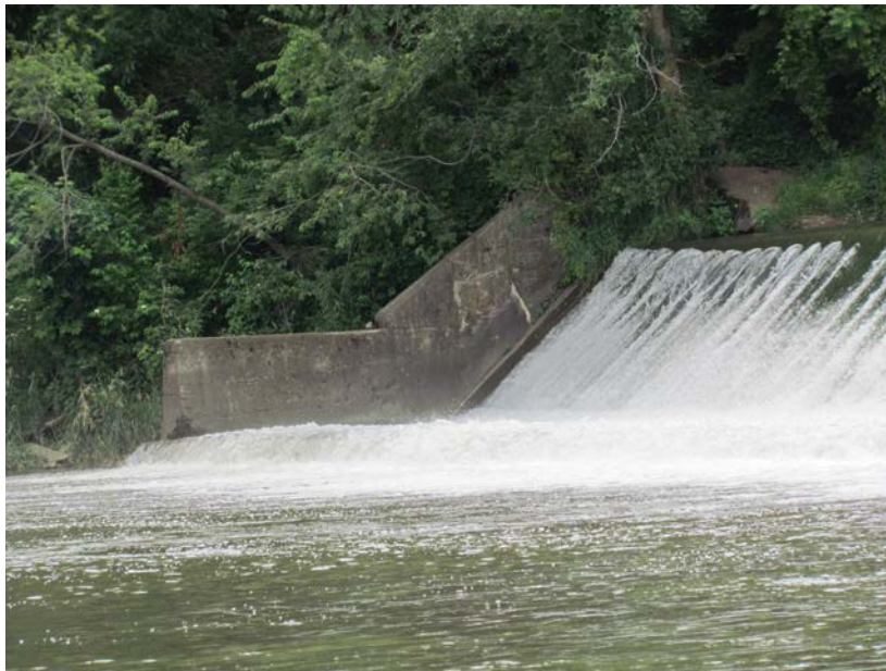
Figure 5. South abutment of the Monticello Electric Company Dam (site 53-00900), near Monticello, Iowa, facing south. Photograph by Richard Carlson, June 23, 2016.
