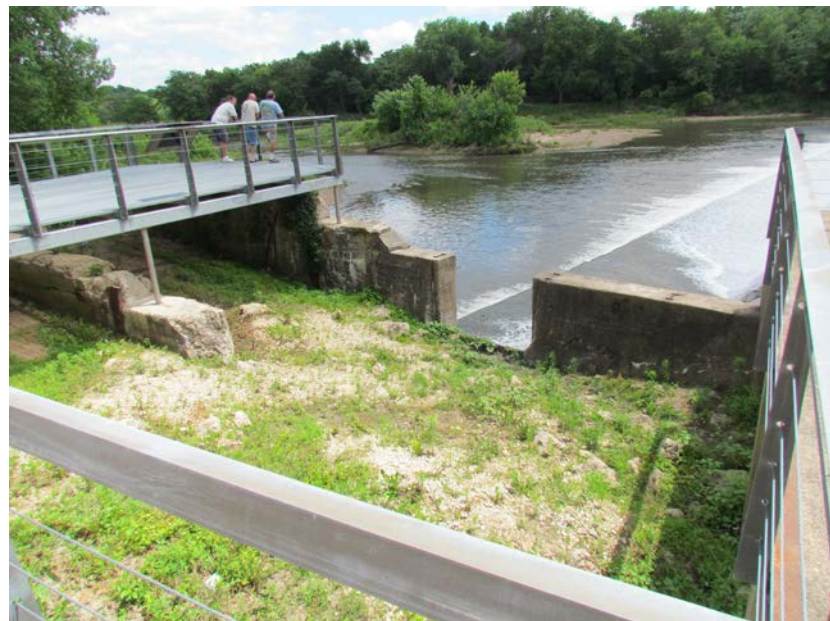
Figure 8. Former race location and north end of the Monticello Electric Company Dam (site 53-00900), near Monticello, Iowa, facing southeast. Photograph by Richard Carlson, June 23, 2016.
