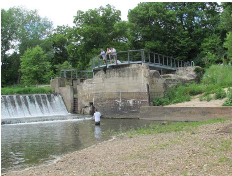
Figure 6. North abutment of the Monticello Electric Company Dam (site 53-00900) and former race wall and powerhouse base, near Monticello, Iowa, facing northwest. Photograph by Richard Carlson, June 23, 2016.
