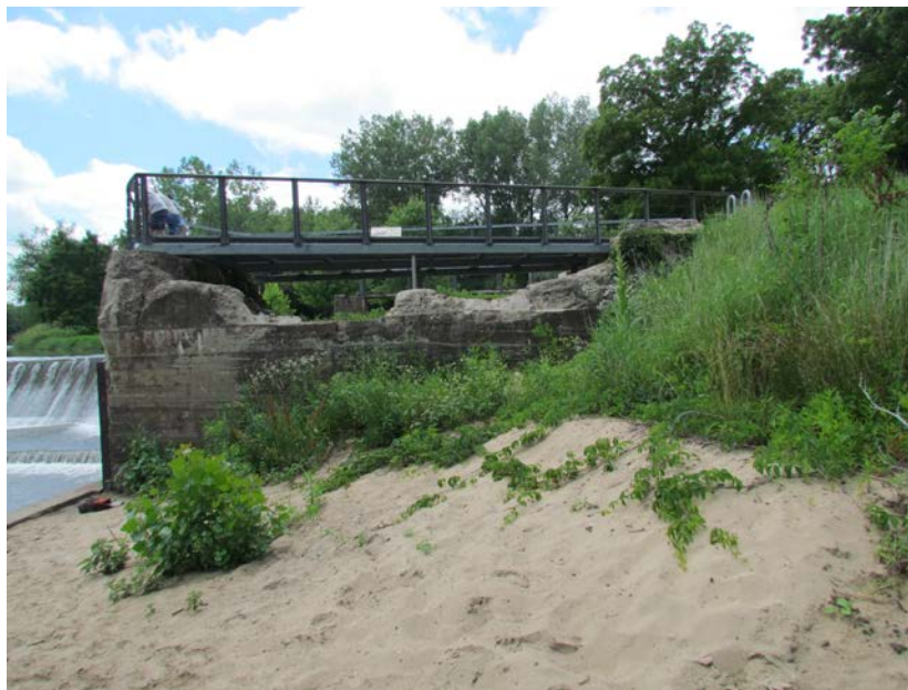
Figure 9. Former race wall and modern observation deck at the Monticello Electric Company Dam (site 53-00900), near Monticello, Iowa, facing southwest. Photograph by Richard Carlson, June 23, 2016.
