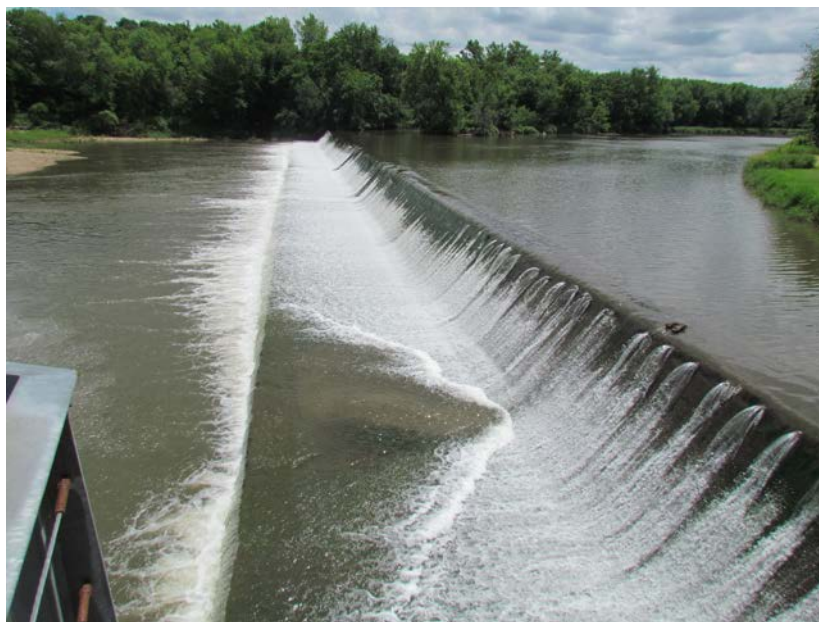
Figure 4. The Monticello Electric Company Dam (site 53-00900), near Monticello, Iowa, facing south-southeast. Photograph by Richard Carlson, June 23, 2016.
