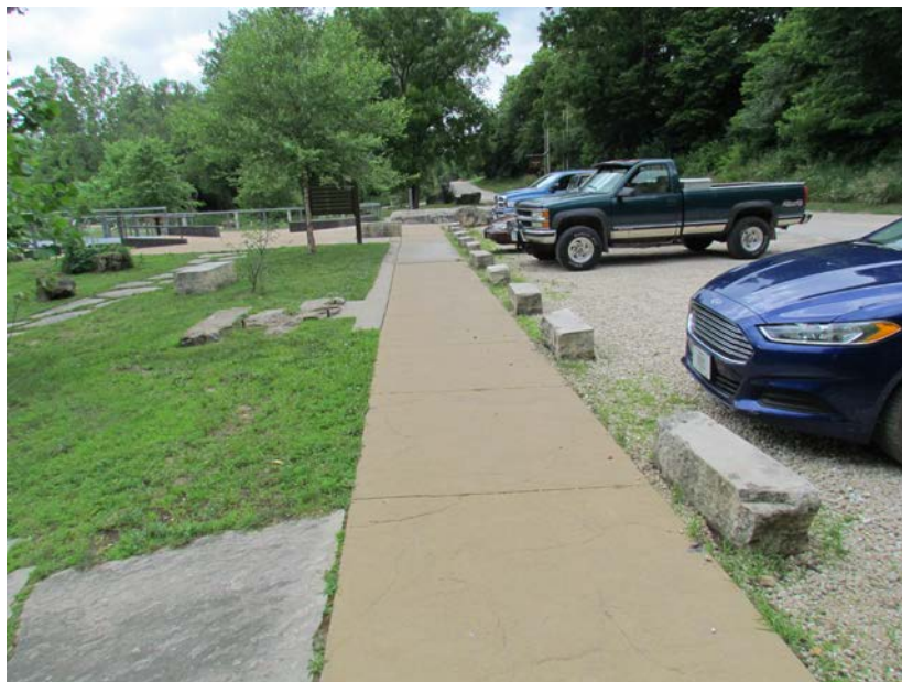
Figure 13. Powerhouse site and parking lot by the Monticello Electric Company Dam (site 53-00900), near Monticello, Iowa, facing southwest. Photograph by Richard Carlson, June 23, 2016.
