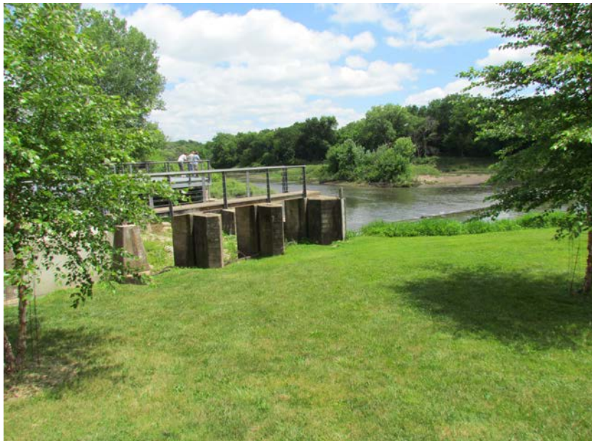
Figure 11. Catwalk and the Monticello Electric Company Dam (site 53-00900), near Monticello, Iowa, facing southeast. Photograph by Richard Carlson, June 23, 2016.
